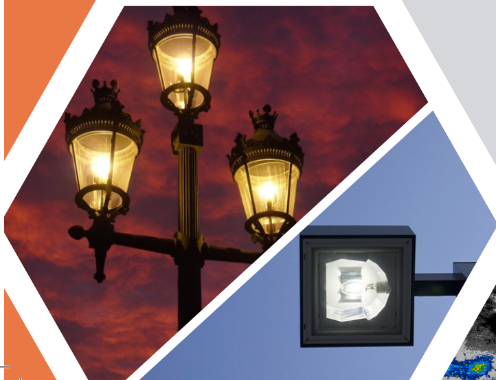
< Fig. 1. An unshielded light fixture (top) as compared to a shielded one (bottom). Half of the light from unshielded fixtures is unproductive, wasting billions of dollars each year.
